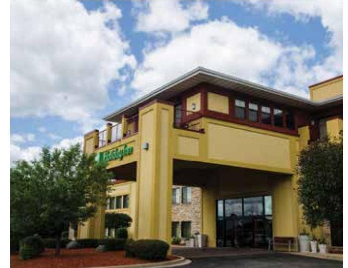
HOLIDAY INN PEWAUKEE-MILWAUKEE WEST N14 W24140 Tower Place, Pewaukee (800) 333-3333 visitwaukesha.org/holiday-inn
